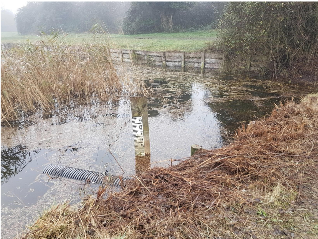
Photo B.3: View of pipe culvert and gauge board at western end of the Cut
