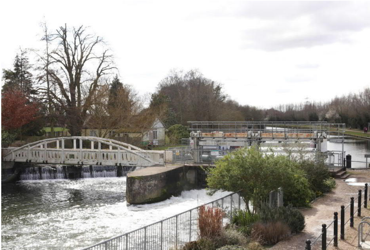
Photo 3: River Cam Corridor LCA – river management infrastructure, sheet piled river banks and the tree-lined towpath are typical features of the area.
